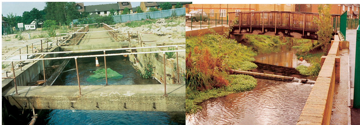
Figure 5: River Wandle at Mill Lane before and after restoration.
